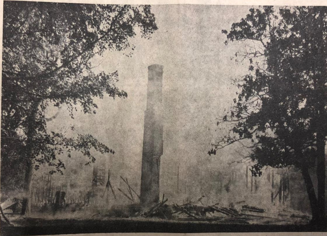
TRAGIC FIRE —All that was left of this home, located on the Dresden Highway, near Ralston, were the chimneys and smoldering ashes. The fire not only burned the home but snuffed out the life of a week old Negro child as well. Fire started from an explosion of a coal oil stove Monday morning.
